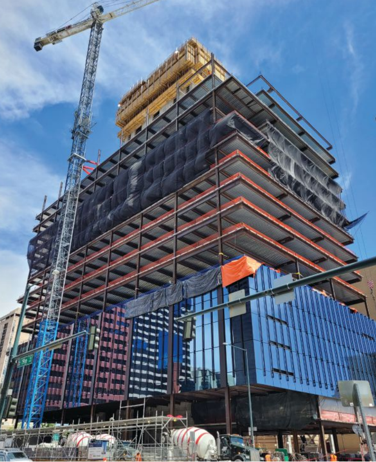
below: Steel framing attaching to the concrete core.
